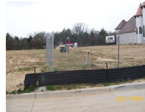
FENCED JOB SITE
