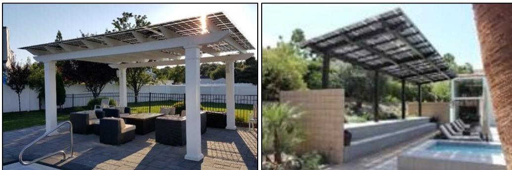
Flat roof mounted on accessory buildings
